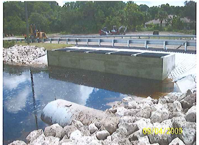
New Water Control Structure #503 on Apollo Waterway
